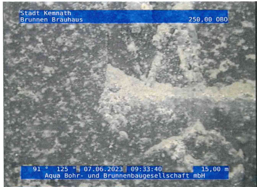
15, 00:13:37, 15.00m OK Filterrohr
